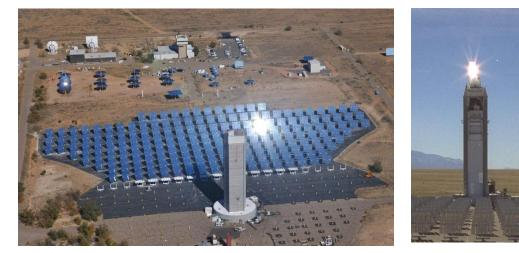
Heliostats and Central Receiver at Sandia Labs, Albuquerque, NM
