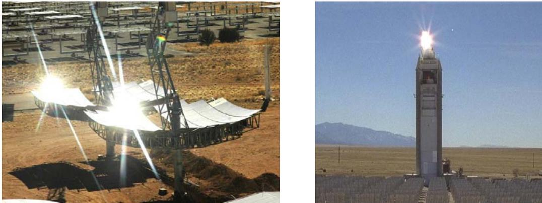
**Figure 1. Examples of specular reflections from mirror facets (left) and diffuse reflections from a central receiver (right).**
