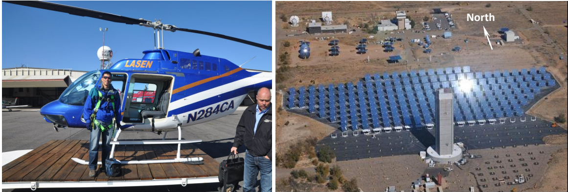
Figure 1. Left: Preparing for a helicopter flyover of the National Solar Thermal Test Facility at Sandia National Laboratories in Albuquerque, NM. Right: Observations of glare from heliostats placed in a standby position aimed ~30 m to the east of the top of the tower (11/10/2010).
